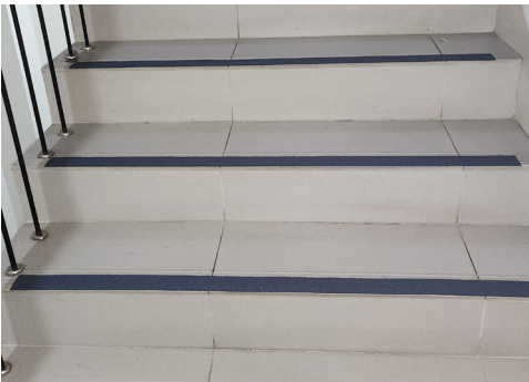
Implementation of non-slip measures on emergency staircases
