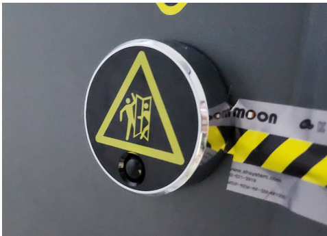
Installation of collision prevention sensors on fire doors
